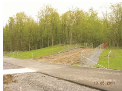
Wildlife fencing is angled backwards because turtles can climb fences
